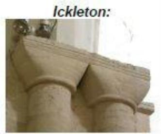
During the 13th-century damage was caused, still visible today, when mouldings were cut away for the installation of altars (SECH, 1994).
